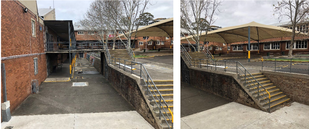
Figure 12. These images, taken from the northeast corner of the existing Liverpool Boys School internal courtyard looking toward the south and southwest, highlight level difference in levels in the LBGHS site.
