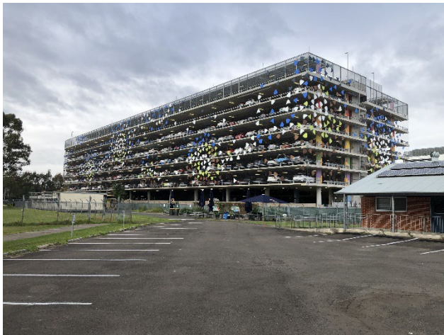
Figure 33. View looking south to Liverpool Hospital carpark (Source: NBRS).
